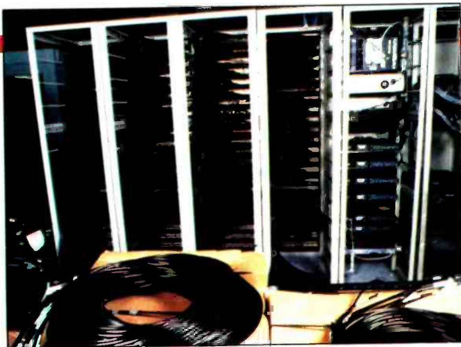
A 200x200 wideband digital routing switcher being installed at Madison Square Garden in New York. Beyond the operational advantages of such a routing system, its physical space requirements are typically less than an equivalent patchbay/DA system would require. (Photo courtesy of BTS.)
