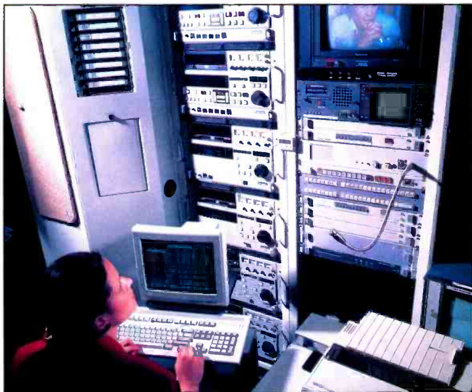
The computer has formed a common interface between operators and many different pieces of broadcast equipment. (Photo courtesy of Odetics.)
