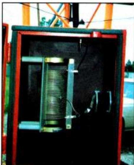
Detuning box containing inductor (left) and capacitor, with base of new tower directly behind. Note detuning skirt wires around tower, terminating at feedthrough insulator on top of box.
